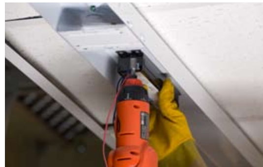
4. Disconnect power from the existing ballast, remove, and recycle.
