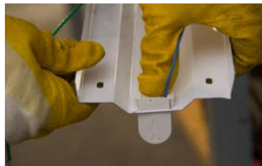
6. Snap in sockets into each end of Ballast Cover .
