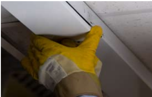
1. Remove existing Ballast Cover .
